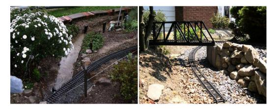
So I put a drain pipe with 3/4 inch holes drilled every 3 inches to drain off the water then I mostly backfilled with driveway stone and topped it off with quarry dust. When it rained again all the quarry dust washed into the driveway stone and became mostly water tight.
